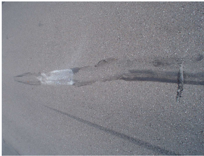
Photo 1: Skid marks on the runway indicate that the pilot must have landed on the nose wheel first
