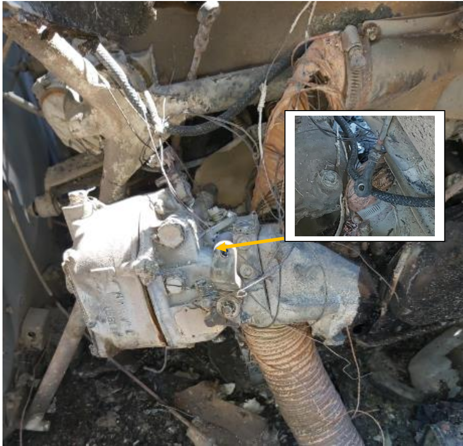
Figure 7: The separated cabrettor throttle control lever and (inset) throttle control cable. (Source: University of Pretoria)
