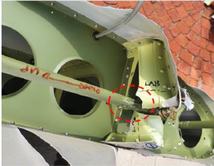
Photo 10: Aileron pushrod impact damages (digital)
