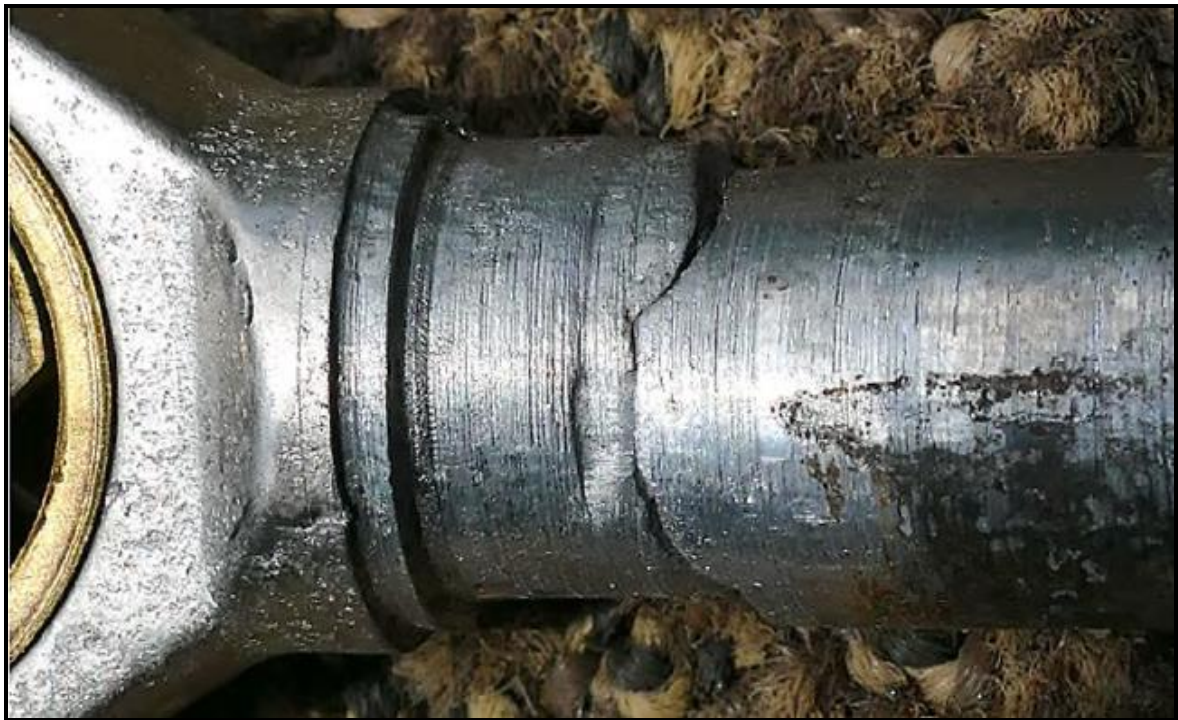
Annexure Figure 14: Shows the failed part of the eye-end bolt
