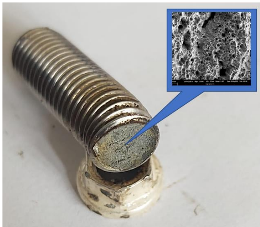
Figure 15: Sheered bolt. (Source: University of Pretoria)
