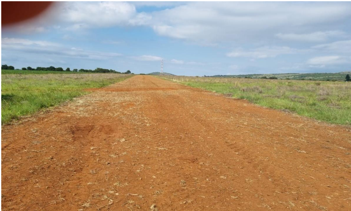
Figure 4: The gravel runway used by the pilot at the farm.
