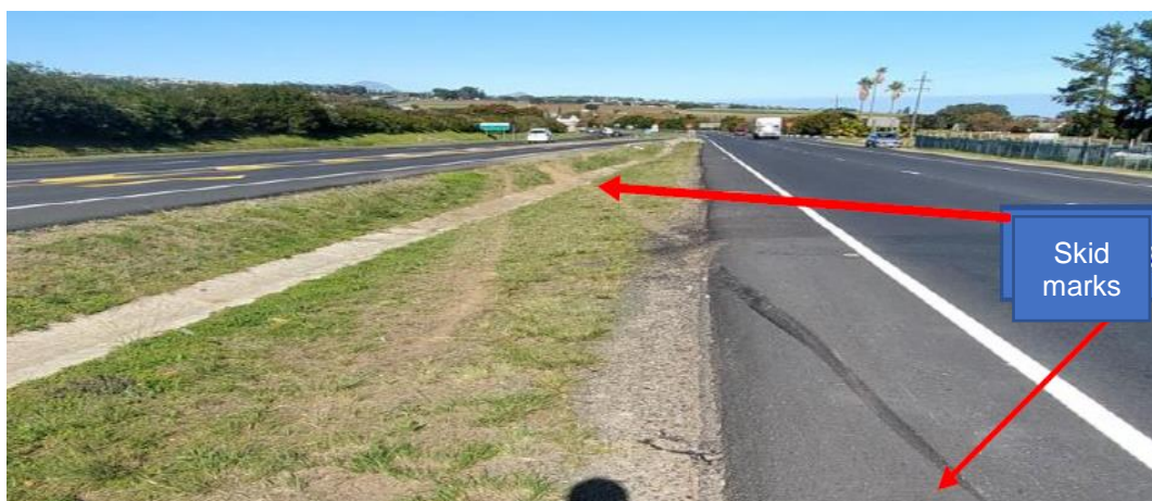
Figure 5: Skid marks on the R44 road and on the dirt centre island.
