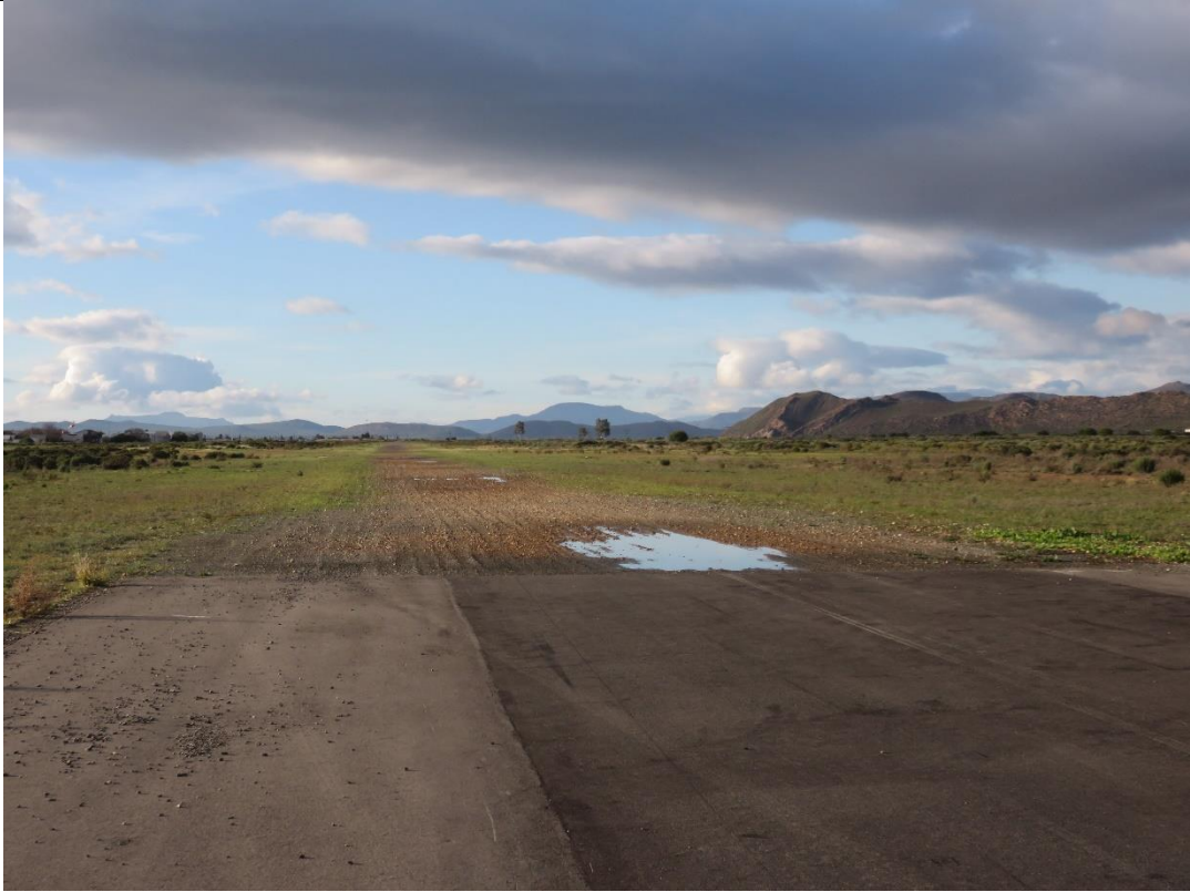
Figure 14: The end of the first asphalt section and the start of the gravel surface.
