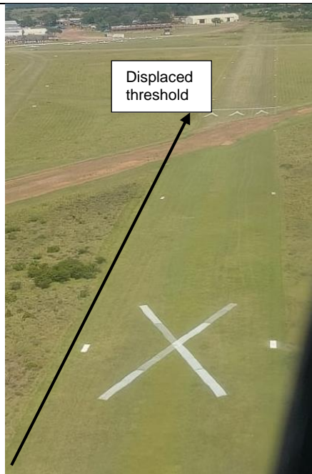
Figure 3: Aerial view of the displaced threshold markings. The arrow shows the length of the displaced threshold. (Source: Airport manager)
