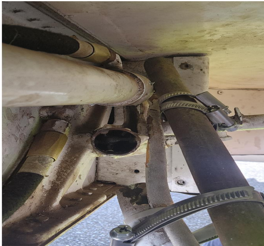
Figure 6: The top part of the drag brace.
