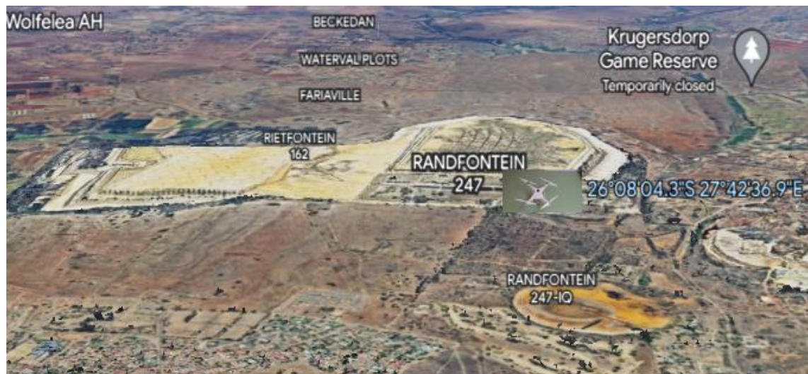
Figure 1: A view of the accident site. (Source: Google Earth)
