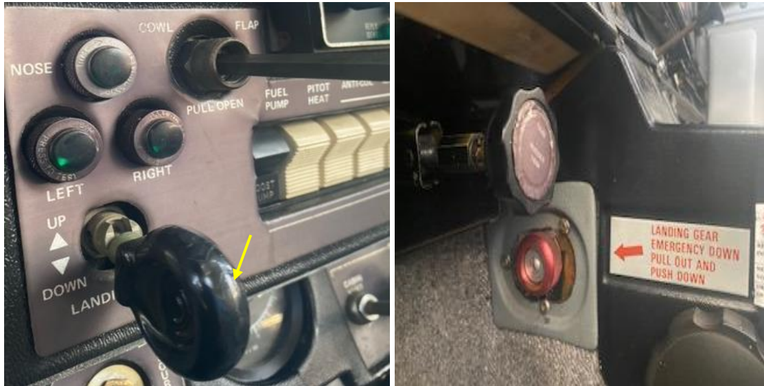
Figures 2 and 3: The gear selector switch/position indicator lights (left). The gear emergency extension (right).
