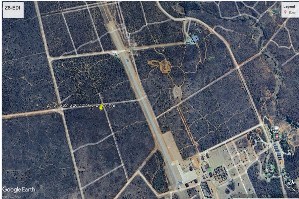
Figure 1: Aerial view of the accident site at Bona-Bona Airstrip. (Source: Google Earth)
