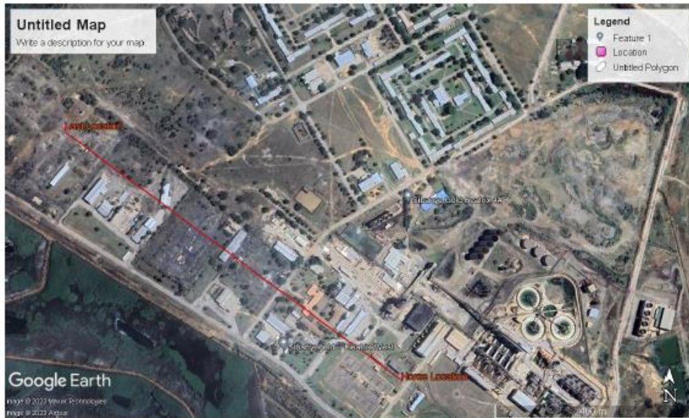
Figure 1: Aerial view of the accident site at Beatrix West Mine (Source: Pilot)
