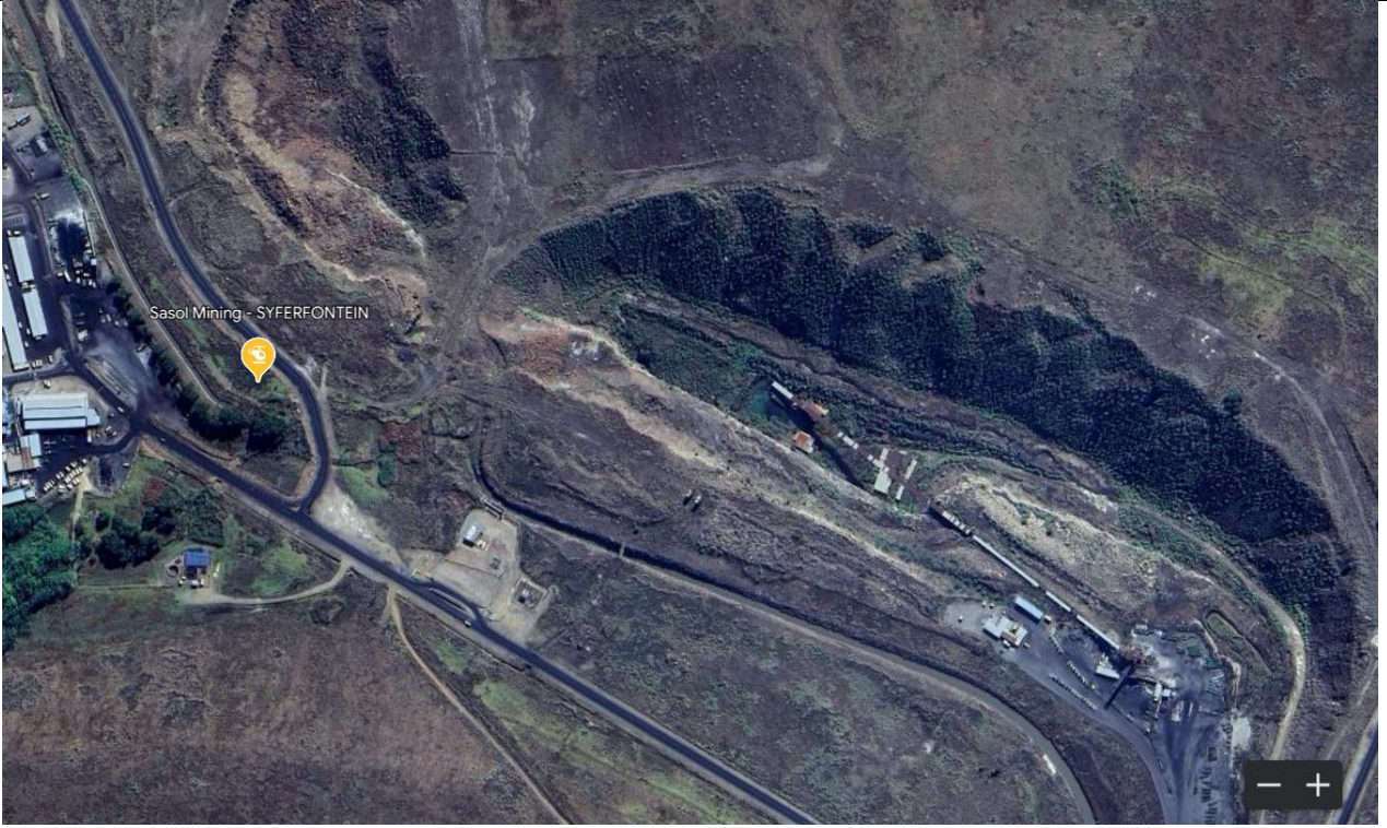
Figure 1: A view of the accident site. (Source: Google Earth)
