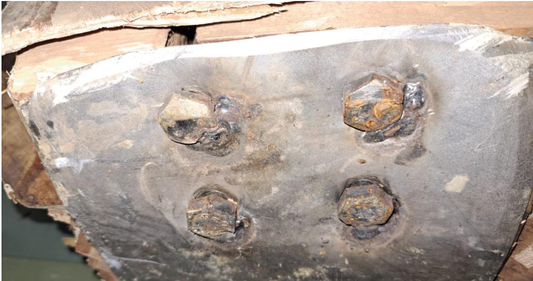
Figure 15: The four-bolt heads welded to the upper support plate (left gear).
