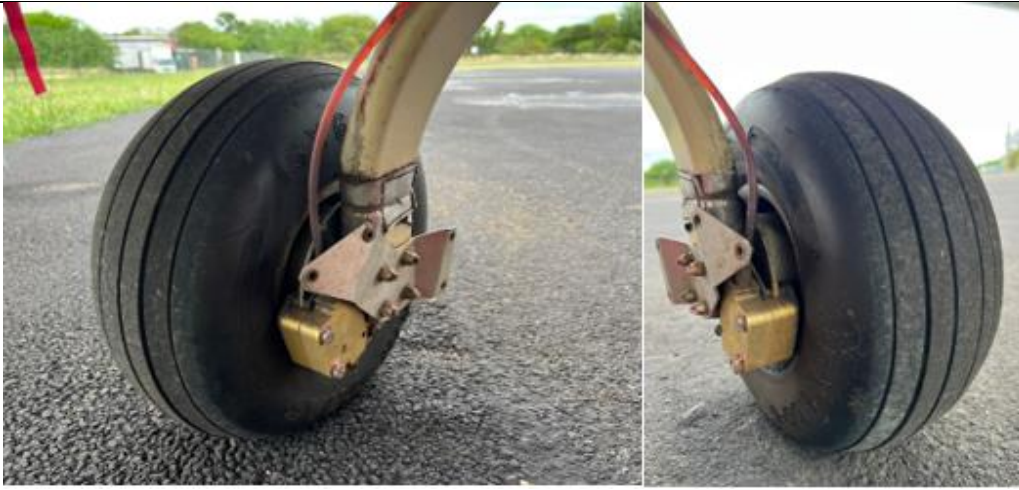
Figure 3: The right and left main landing gear brake pipelings showed no leakage. (Source: AMO)
