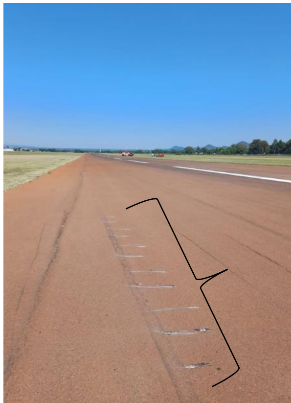
Figure 3: The propeller strike marks on the runway. (Source: Operator)
