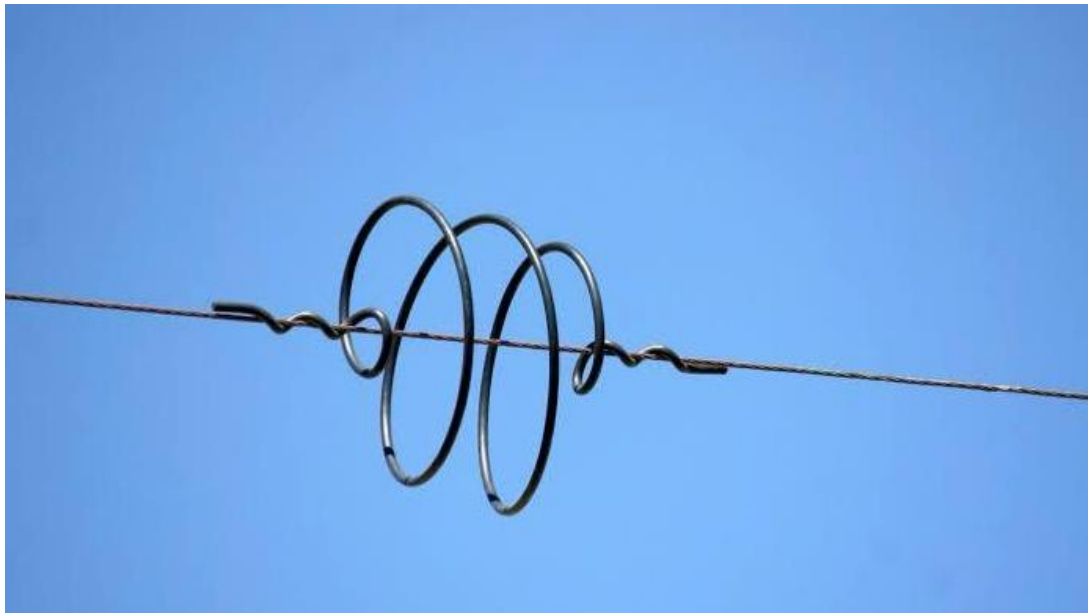
Figure 6: A typical bird diverter fitted on an earth conductor. (Source: https://issuu.com/travelnewsnamibia/docs/conservation_2022_digital_pre/s/17459810 )
