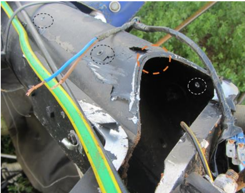
Figure 4: The repair scheme conducted after the incident on 7 February 1987.
