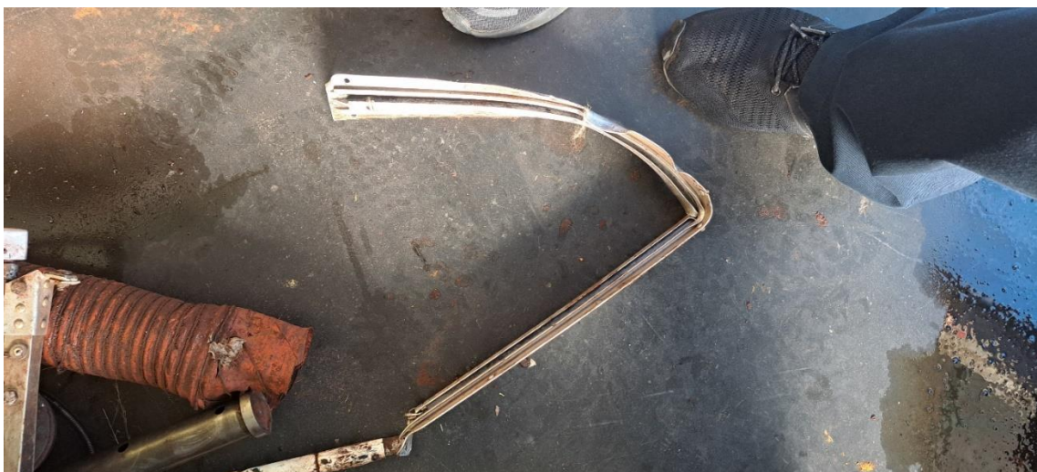
Figure 6: One of the railings that had detached from the airframe with forward bent signature beyond 90°.
