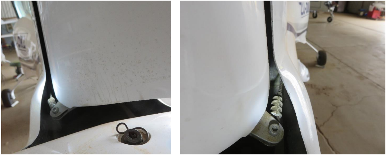
Figure 5(a) and 5(b): The left and right rudder cable connections (rudder side) were found intact.
