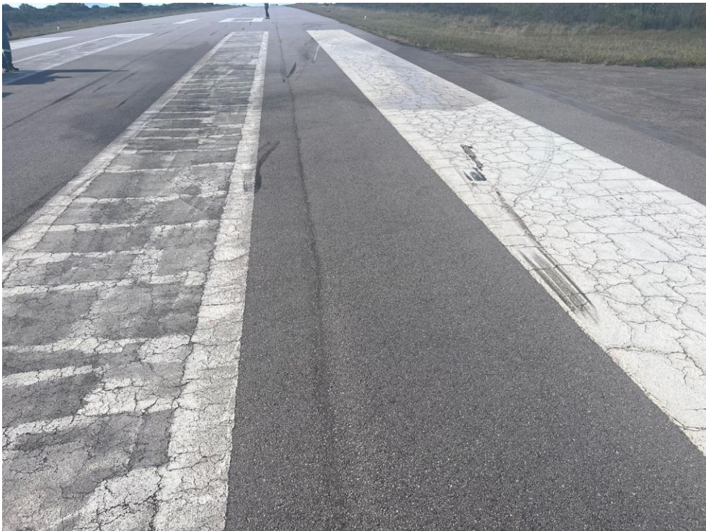
Figure 2: The accident aircraft skid marks on Runway 10 at FAMO. (Source: Owner)
