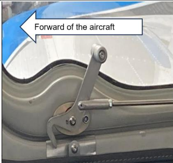
Figure 7: Improperly latched interior door handle.
