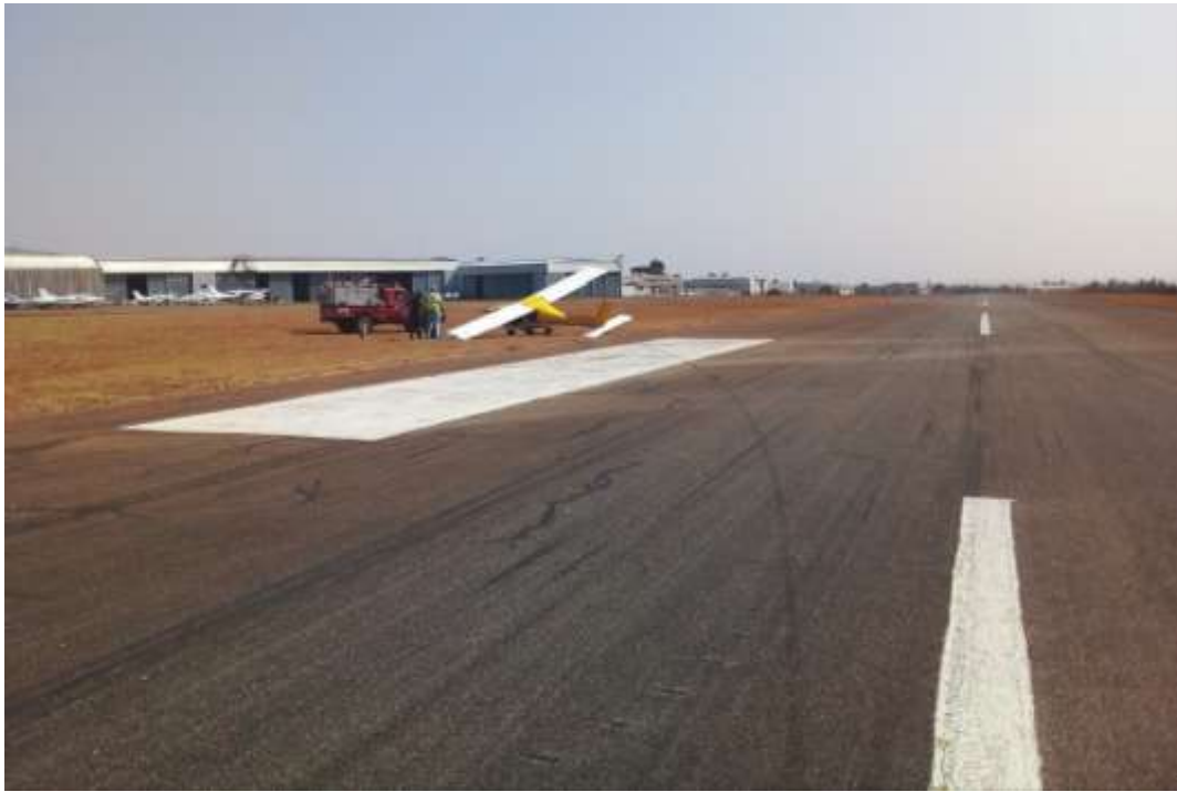
Figure 2: The left main tyre markings on the runway. (Source: Pilot)
