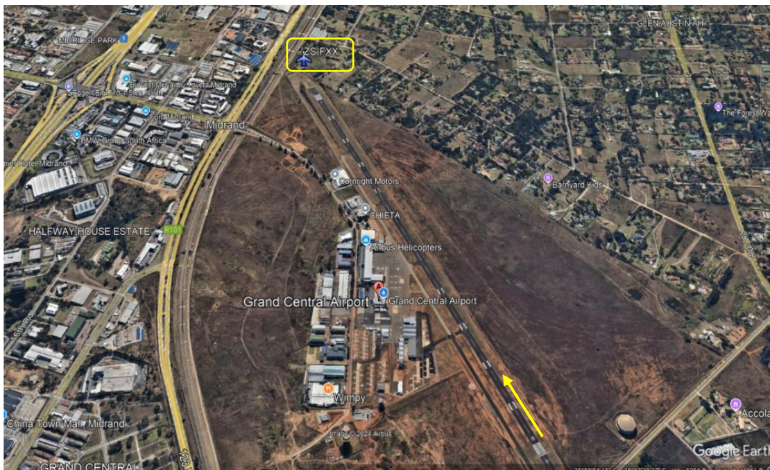
Figure 1: The layout of FAGC, the direction of landing (yellow arrow) and the approximate accident site (yellow rectangle). (Source: Google Earth)
