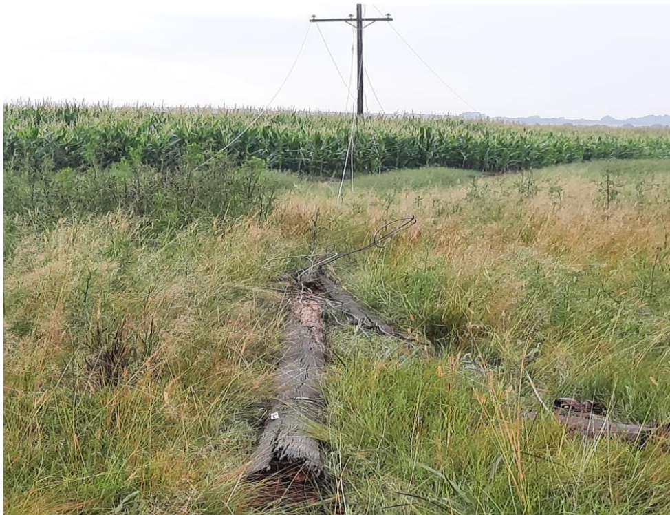
Figure 2: A damaged pole that secured the powerlines after the accident. (Source: Pilot)
