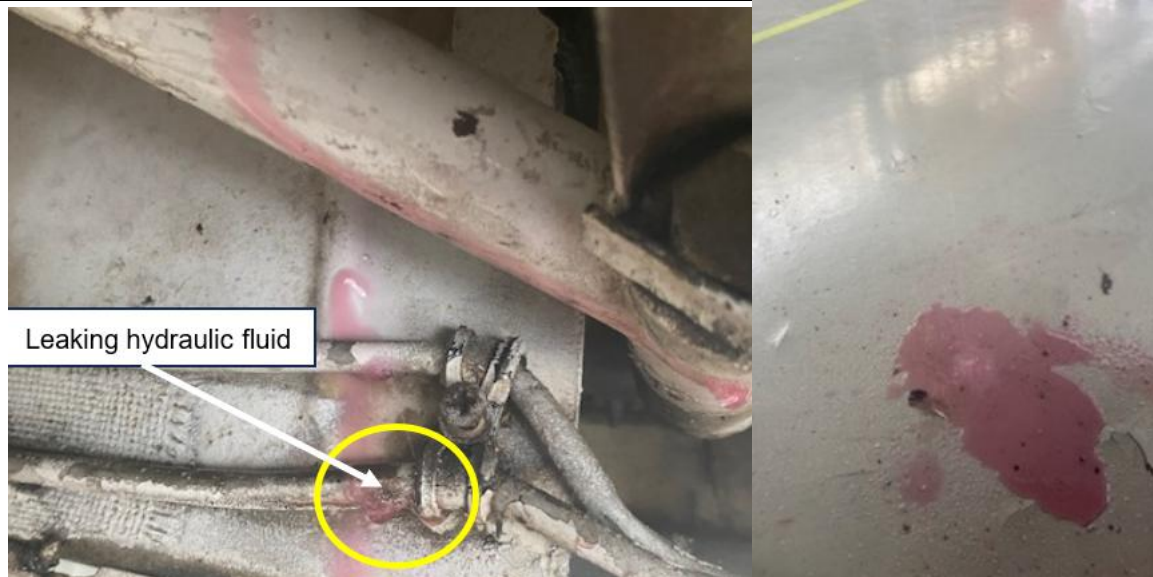
Figure 5: The yellow circle indicates a leak on the hydraulic retraction pipe.
