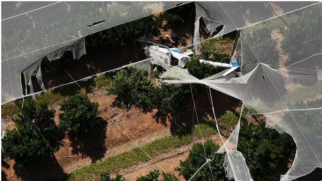
Figure 4: A closer view of the damaged netting and the helicopter.
