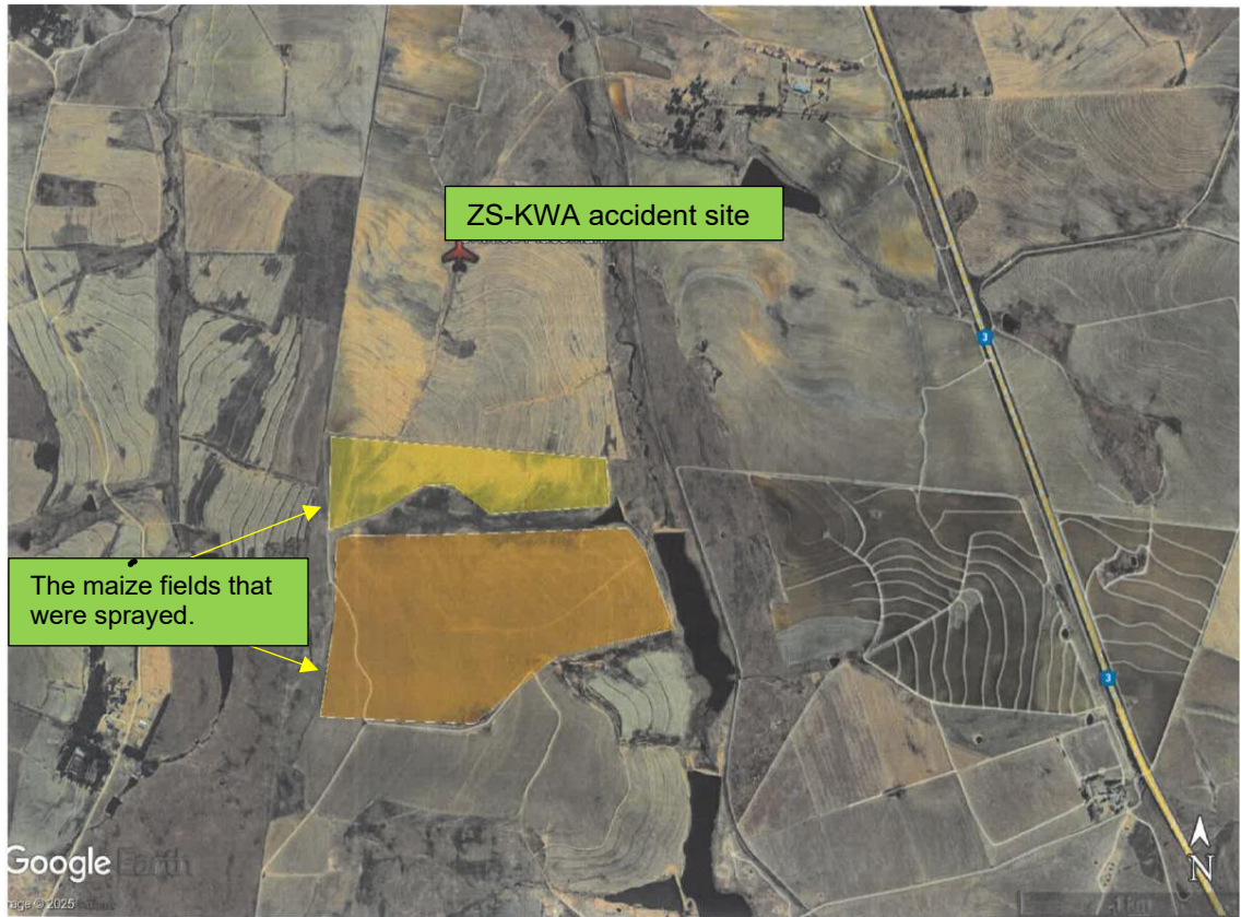
Figure 1: The maize fields that were sprayed and the approximate accident site. (Source: Google Earth)
