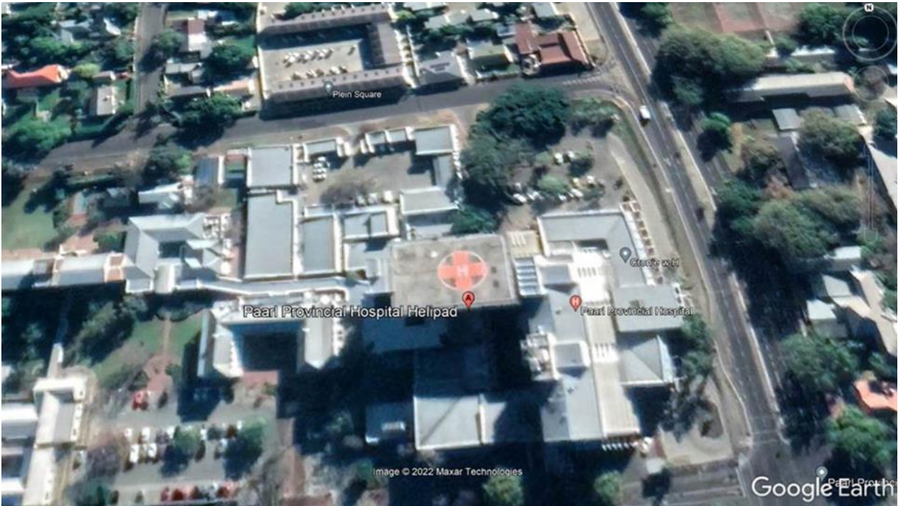
Figure 1: The rooftop helistop where the serious incident occurred. (Source: Google Earth)
