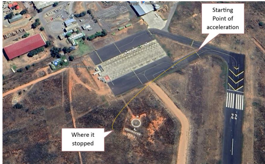
Figure 3: Bird's eye view of the incident site. (Source: Google Earth)
