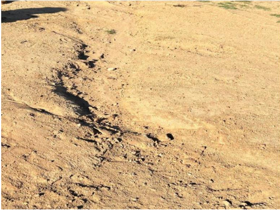
Figure 3: The furrow on the gravel runway caused by rain. (Source: Pilot)
