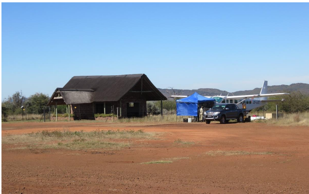
Figure 9: The terminal building with ZS-LEC parked next to it.
