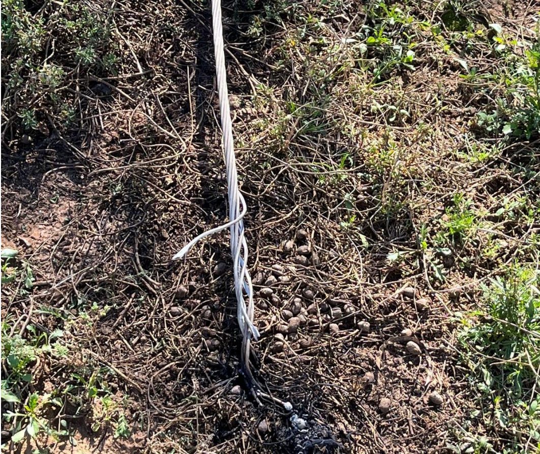
Figure 4: One of the severed cables. (Source: Pilot)
