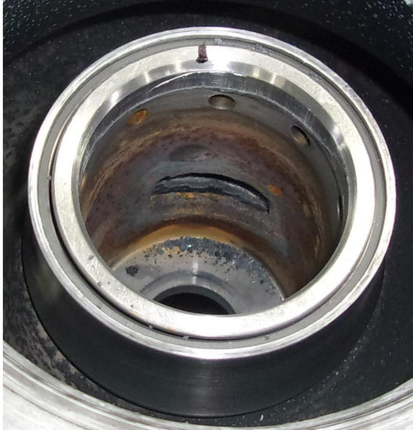
Figure 13: The inside of the turbine end shaft with a hole that had developed at the point of failure of the turbine end journal bearing. The hole had formed at the tip of the bulge due to the heat generated by contact between the rotating shaft and the stationary parts.
