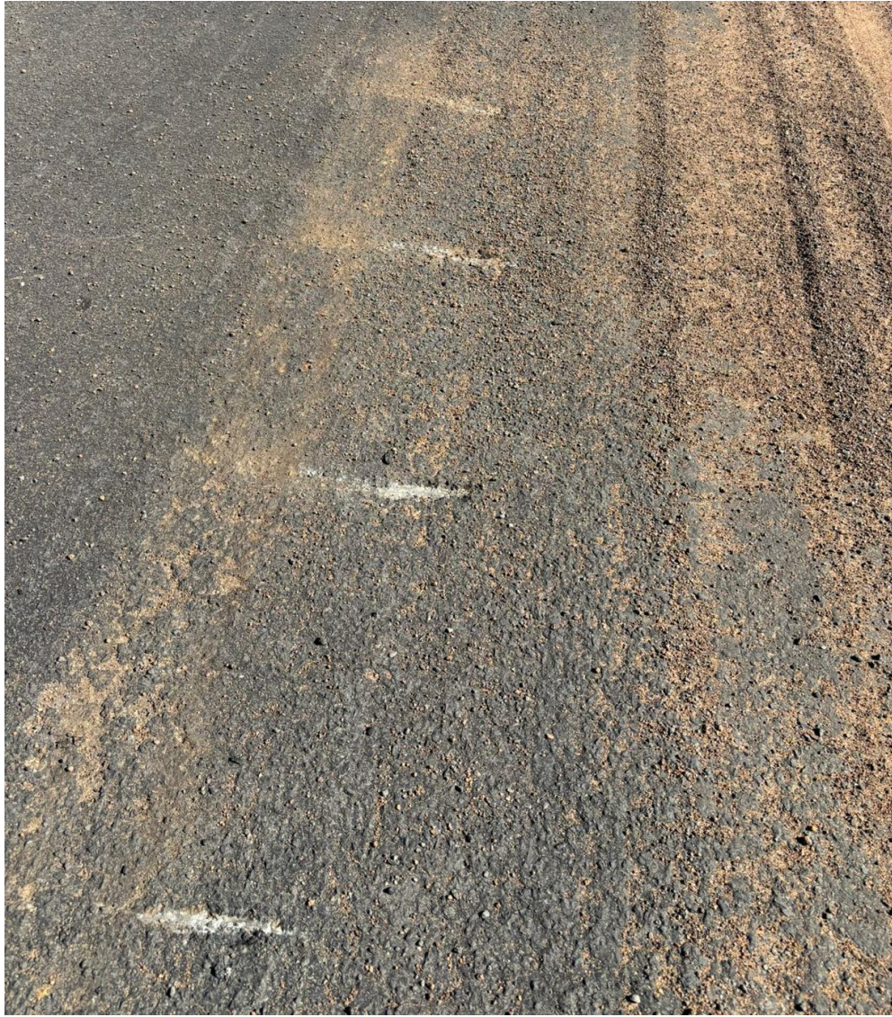
Figure 2: Propeller strike marks on the runway. (Source Pilot)
