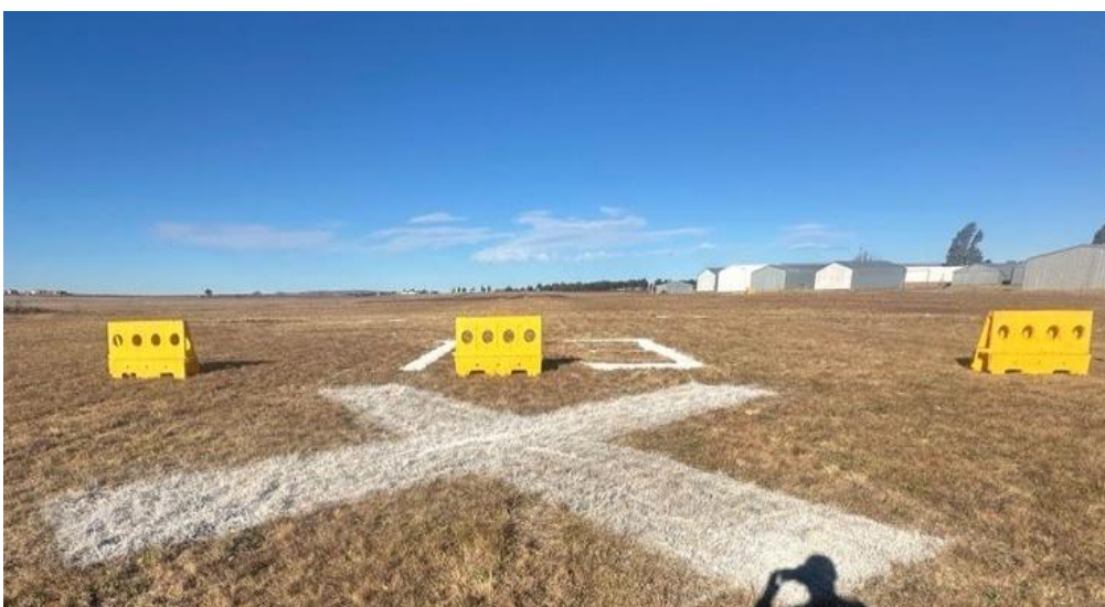
Figure 3: Temporary closure markings on RWY 13 after the serious incident. (Source: Aerodrome manager)
