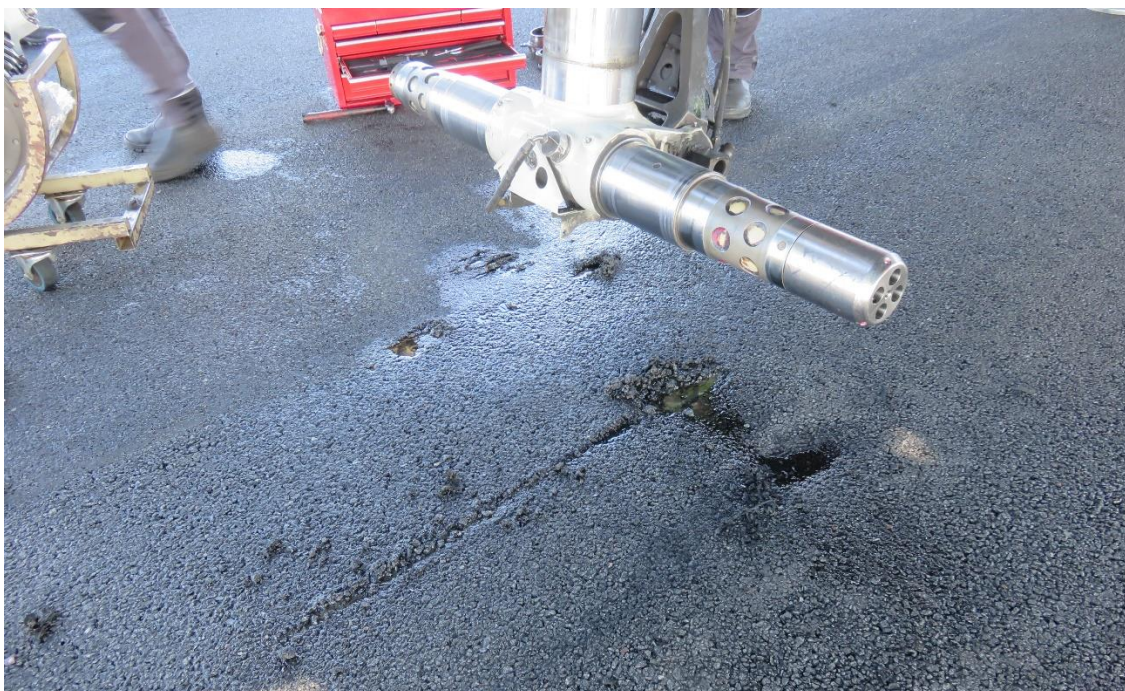
Figure 4: Damage to the runway surface where the aircraft had stopped.
