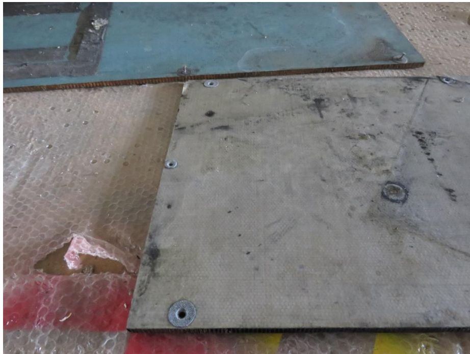
Figure 3: Floor boards damaged by the spilt chemical.
