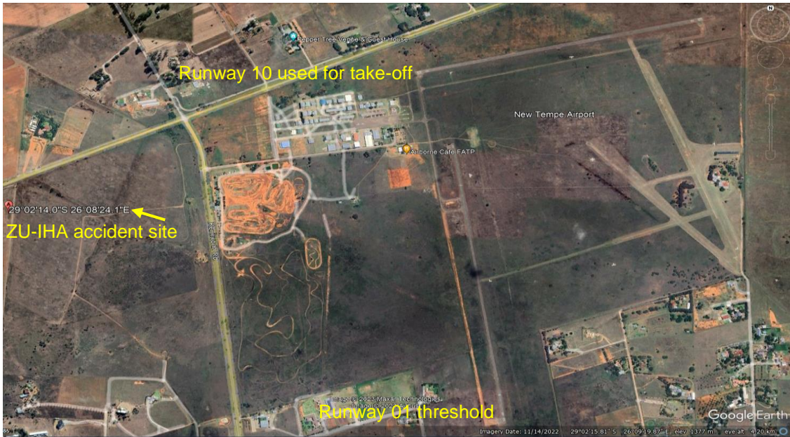
Figure 2: The view of the accident site and the runway used for take-off. (Source: Google Earth Map)
