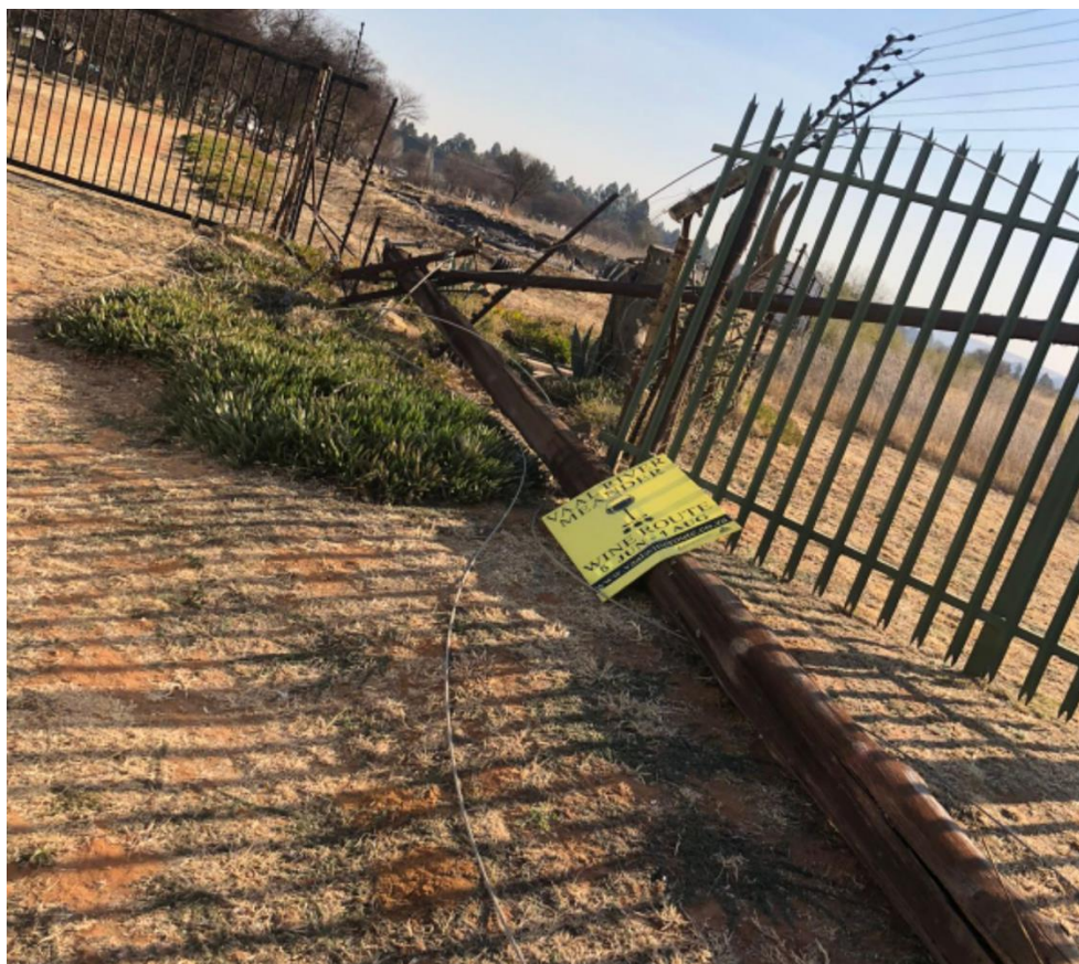
Figure 1: Broken electric pole and damaged palisade fence caused by the collision of the aircraft with the powerlines. (Source: Airstrip owner)
