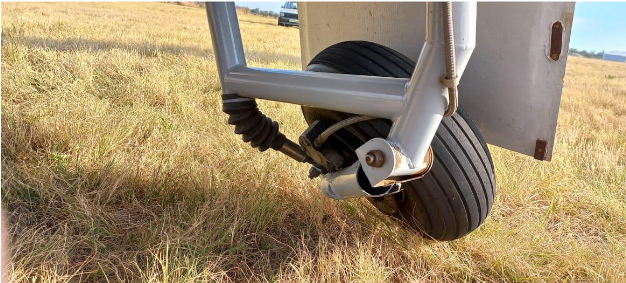
Figure 1: Damage on the left main gear.
