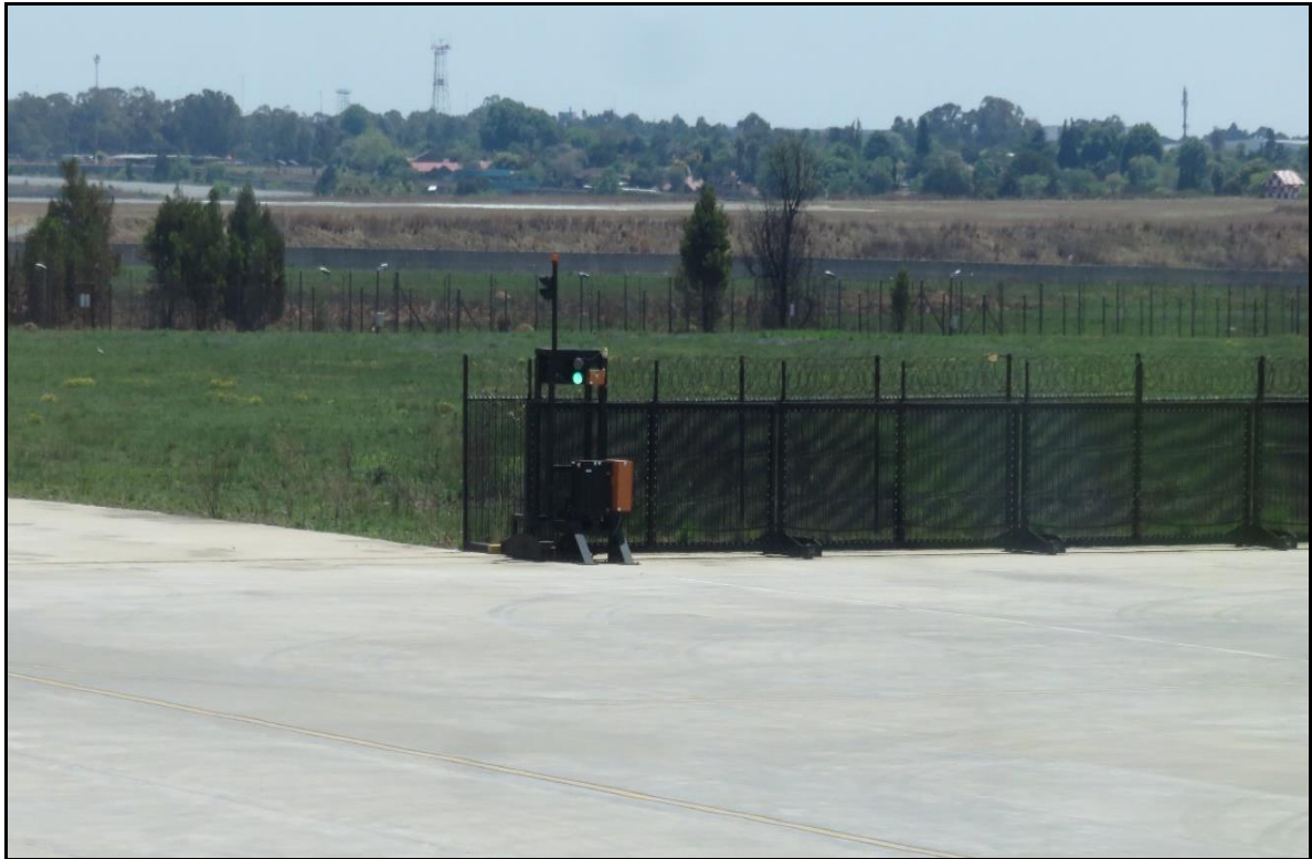
Figure 22: The FBO apron gate and the visible traffic light (illuminating green).
