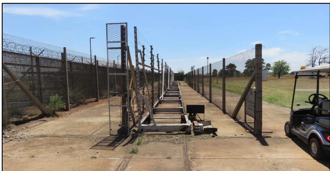
Figure 12: The Denel Campus gate remains in the fully open position.
