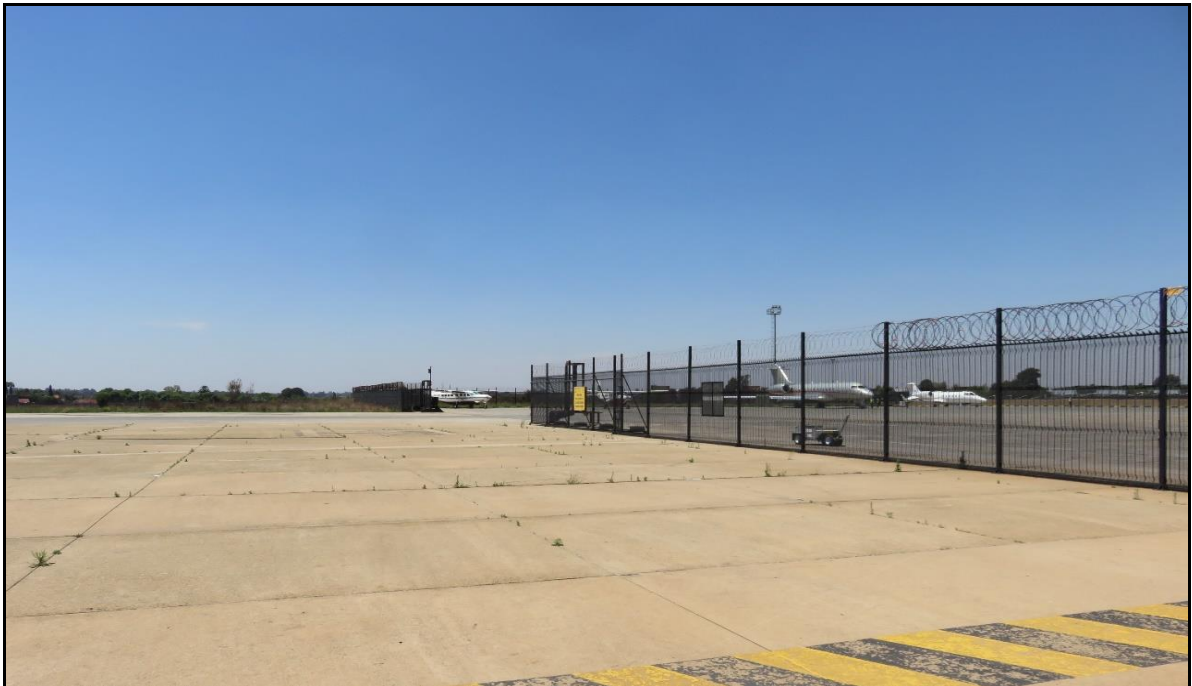
Figure 20: The FBO fenced off area and the gate view from the Denel Campus side.
