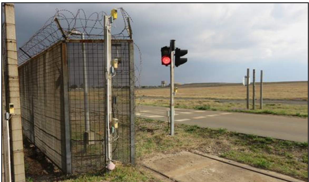
Figure 19: The ACSA/Echo gate traffic light in the gate 'close' position.
