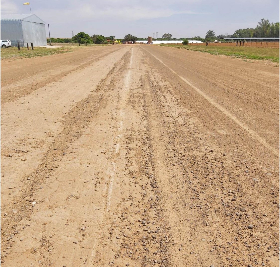
Figure 2: Tyre brake markings visible on the gravel runway.
