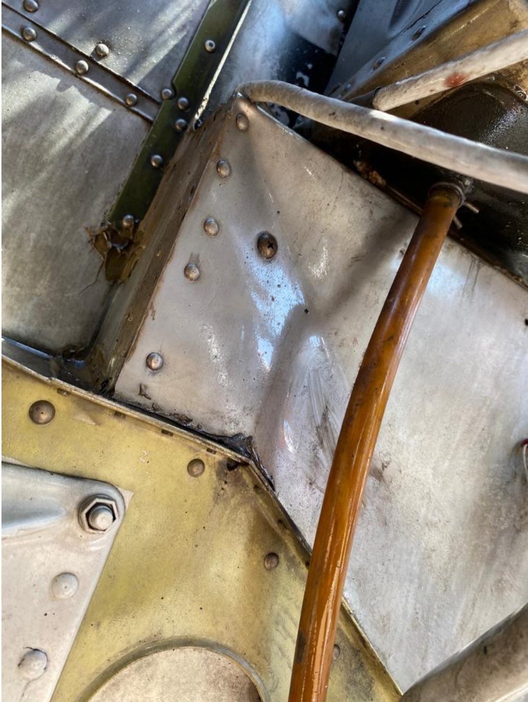
Figure 2: Deformation on the firewall.
