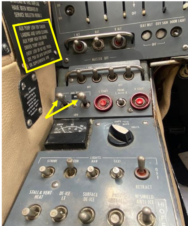
Figure 10: A view of the auxiliary fuel pumps in a HIGH mode setting. There is a placard (yellow window above) installed on the left pilot's side panel stating AUX PUMP HIGH FOR ENGINE DRIVEN PUMP FAILURE (VERY LOW OR NO FUEL PRESSURE).
