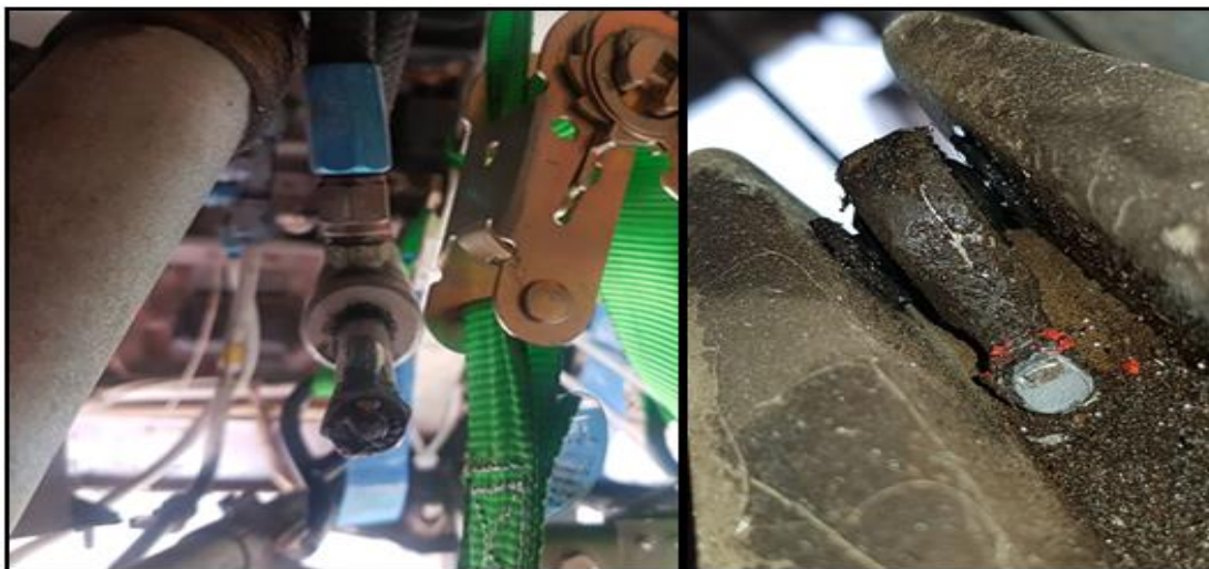
Figure 1: Retraction and extension actuator failure on the bottom connecting rod end (left) and the bearing (right).
