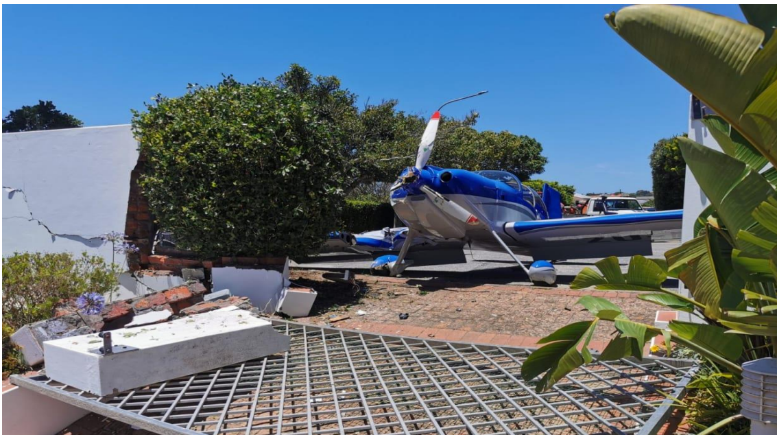
Figure 3: Damaged perimeter wall and motorised access gate. (Source: Fire Chief).
