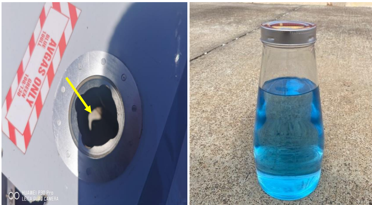
Figures 5 and 6: Dry/empty left tank (left picture). Unusable fuel drained from the left tank drain valve post-accident in a one litre bottle. (Source: Fire Station Chief)
