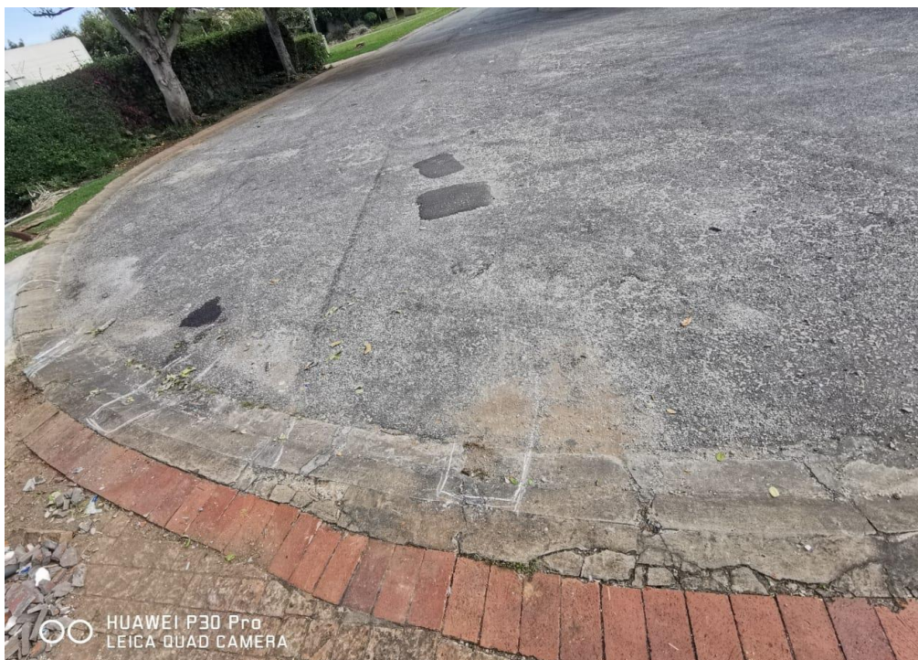
Figure 8: The tarred Erica PI Drive post-accident showing no evidence of fuel spillage. (Source: Fire Station Chief)
