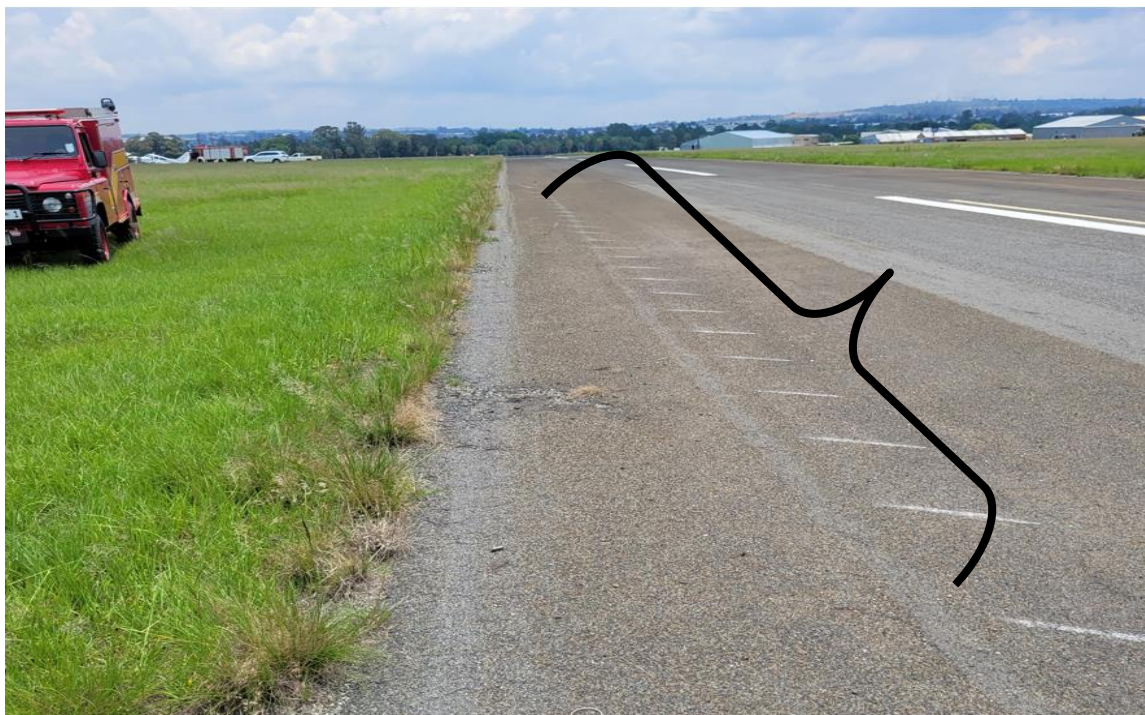
Figure 9: Propeller marks on the runway.
